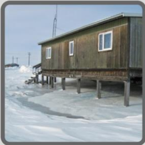
PONDING DUE TO THAW SETTLEMENT
