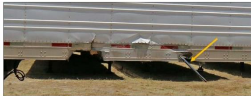
Figure 7. Closeup view of impact damage to the right side of the Utility semitrailer. The arrow indicates a segment of front windshield trim from the Tesla entrapped in the forward-most area of damage.
