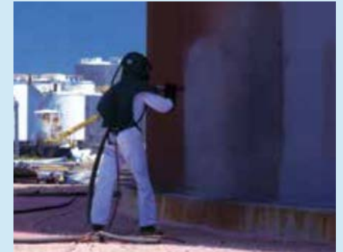
Blasting with garnet significantly reduces dust exposure
