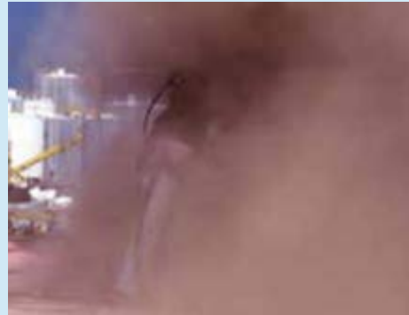
Blasting with conventional abrasives can create excessive dust
