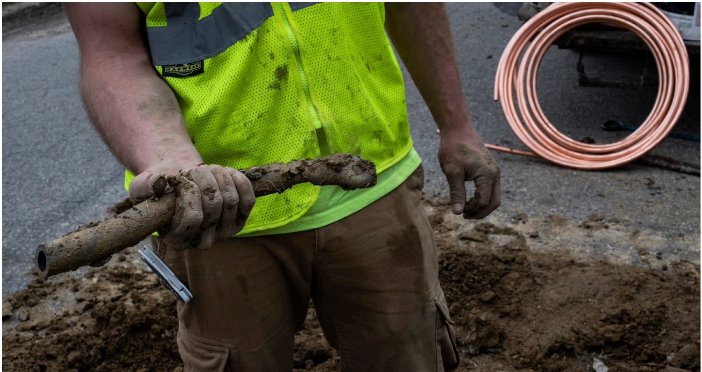
A piece of lead pipe removed during a service line replacement in Flint, Michigan.
