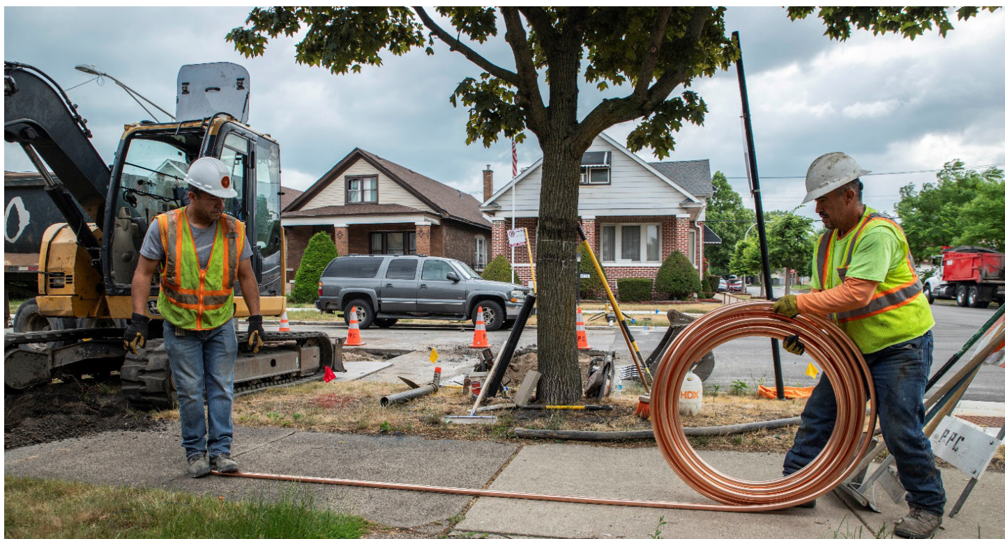
Workers unrolling new copper line outside a home in Chicago, Illinois.
