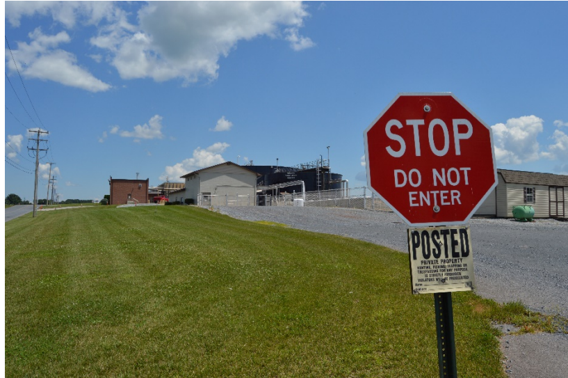
The Keystone Protein Company meat processing plant in Fredericksburg, Pennsylvania, violated its water discharge permit 62 times between January 1, 2016, and June 30, 2018, discharging excessive amounts of nitrogen pollution into a tributary to the Susquehanna River and Chesapeake Bay.
