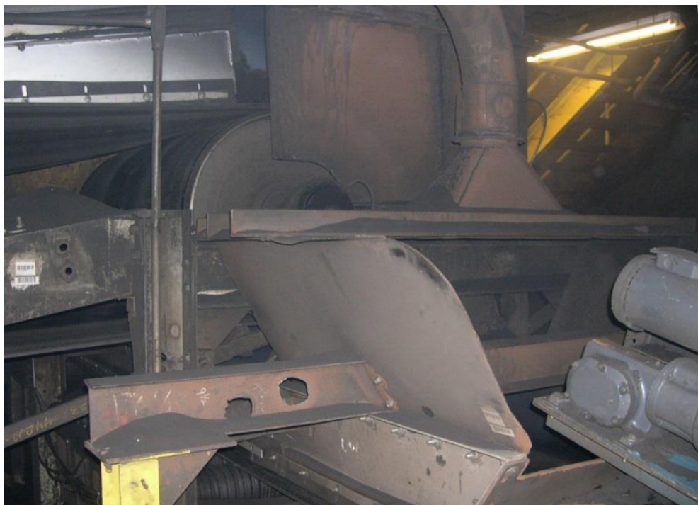
Cleaning Sand Out of Tightly-Compacted Machinery Where Access is Extremely Limited
