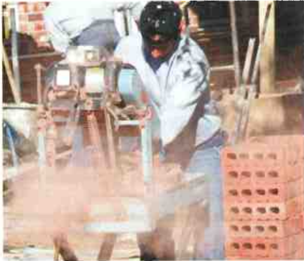
Using a stationary masonry saw without dust controls can expose workers to high levels of silica. Table 1 provides a simple explanation of what employers can do to keep their workers safe. (Photo courtesy of CPWR)
