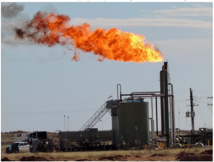
A malfunctioning flare at a tank battery in the New Mexico Permian Basin, photographed on Feb. 6, 2023. Incomplete combustion in a flare, as pictured, generates more emissions. Credit: WildEarth Guardians
