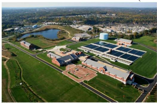
became operational in 2006, replacing three older treatment plants that were unable to meet the requirements of the D/DBP rule. Conventional treatment processes with the addition of ozone and biologically active carbon filtration were chosen for the Griffith Plant to meet D/DBP rules. An initial evaluation by engineering consultants has determined that additional treatment trains are necessary to remove PFOA and PFOS to the proposed MCL.
