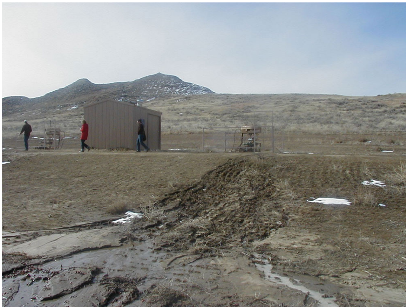
This coal-bed methane gas well in the Powder River Basin leaked water, which caused some erosion. The facility was abandoned by its operator, and the state later plugged the well and reclaimed the area. (Courtesy of Jill Morrison — click to view )
