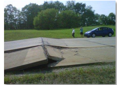
Roadways in the Upper Midwest are susceptible to freeze-thaw damage in the winter months (left) and expansion buckling during summer heat (right). Changes in winter impacts to roads are uncertain, but damage from heat may be more probable with an increasing number of hot days. Photos: AP
