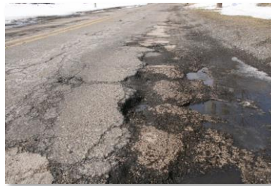
Roadways in the Upper Midwest are susceptible to freeze-thaw damage in the winter months (left) and expansion buckling during summer heat (right). Changes in winter impacts to roads are uncertain, but damage from heat may be more probable with an increasing number of hot days. Photos: AP
