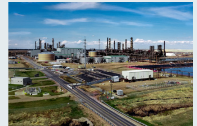
Sturgeon Refinery Aerial. Image courtesy of Alberta Carbon Trunk Line.
