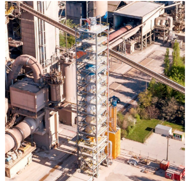
Calix advanced calcination reactor at their LEILAC pilot plant in Belgium. Image courtesy of Calix.
